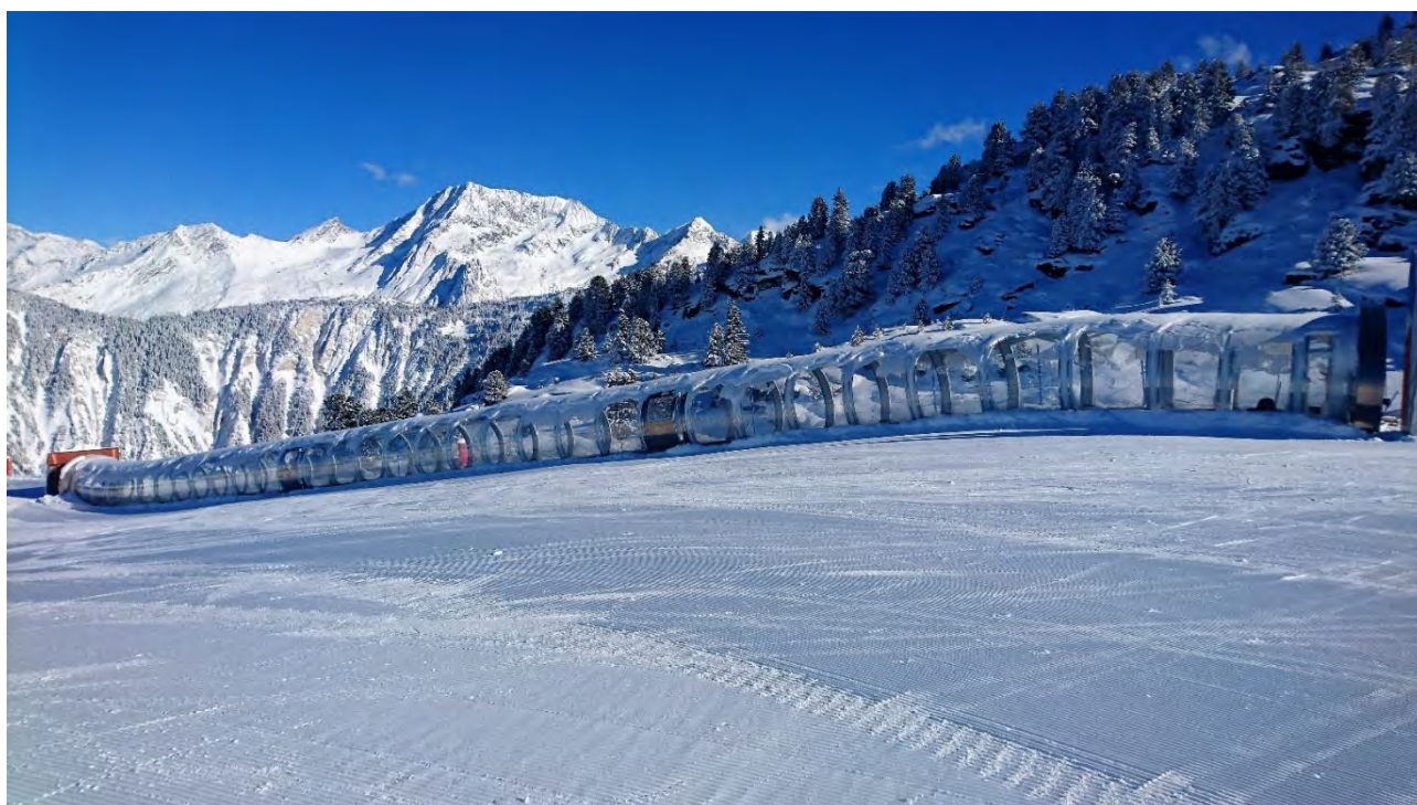
2016 - Chourchevel (France) – Length 68 m – Band width 600 mm
