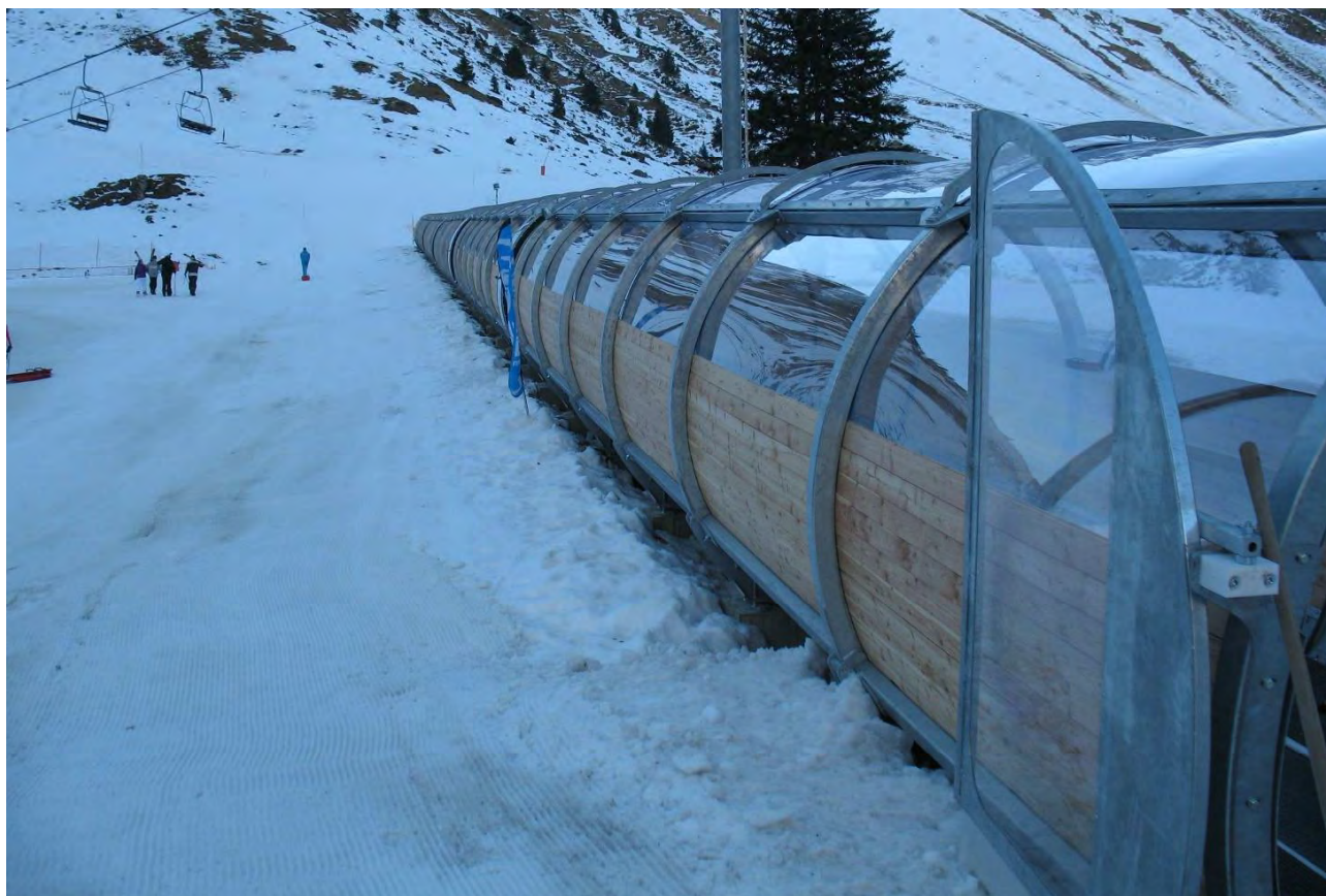
2015 - Barèges (France) - Canopy with wood siding – Length 120 m – Band width 600 mm
