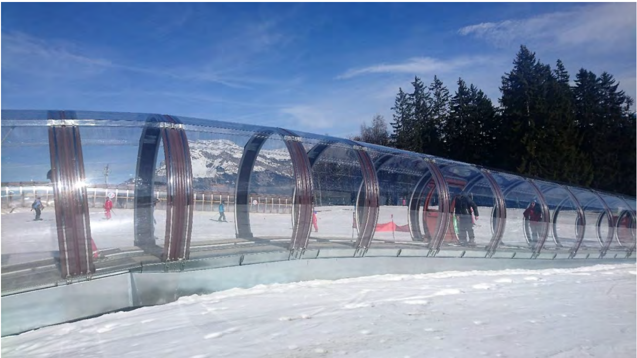
Side view of the MND Ropeways canopy
