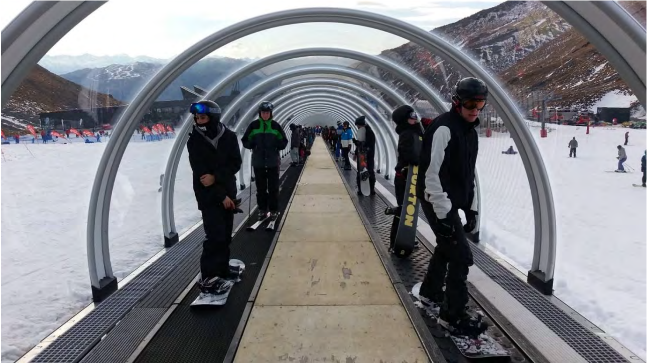
2017 – Remarkables (New Zealand) – Length 160 m – Large canopy to cover 2 existing conveyors
